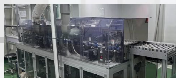
4. cell纯水清洗 Cell Deionized Water Cleaning
